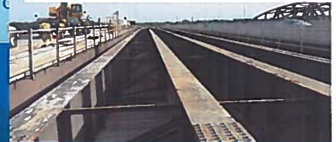
1960'S STEEL STRINGERS REMOVAL
