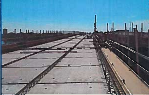
New Concrete Deck Panels
